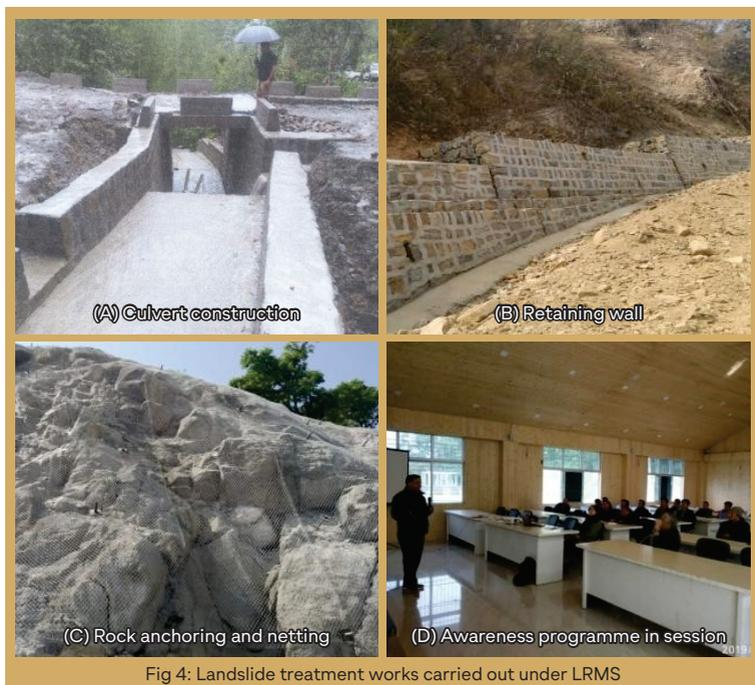
Fig 4: Landslide treatment works carried out under LRMS
